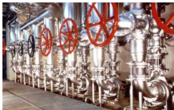
Pump station with vibration absorbers
