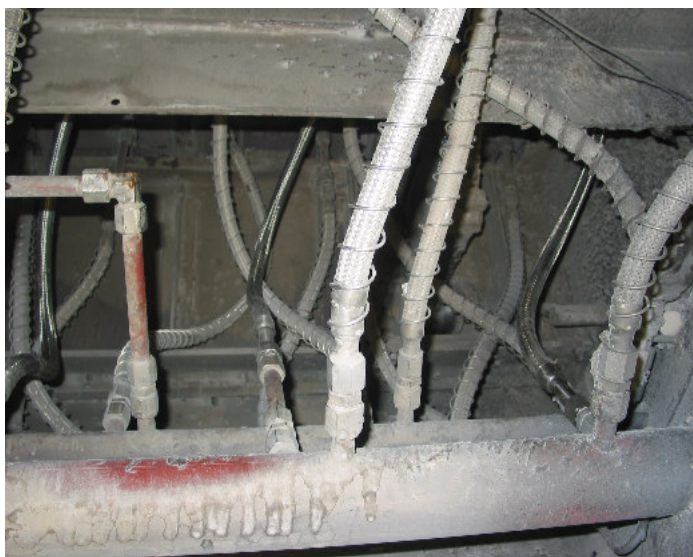
Use of metal hoses in a waste incineration plant
