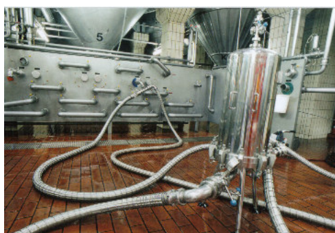
Use of a metal hose assembly in a brewery
